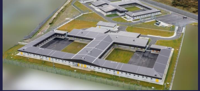
Christchurch Men Prison – Modular Project
